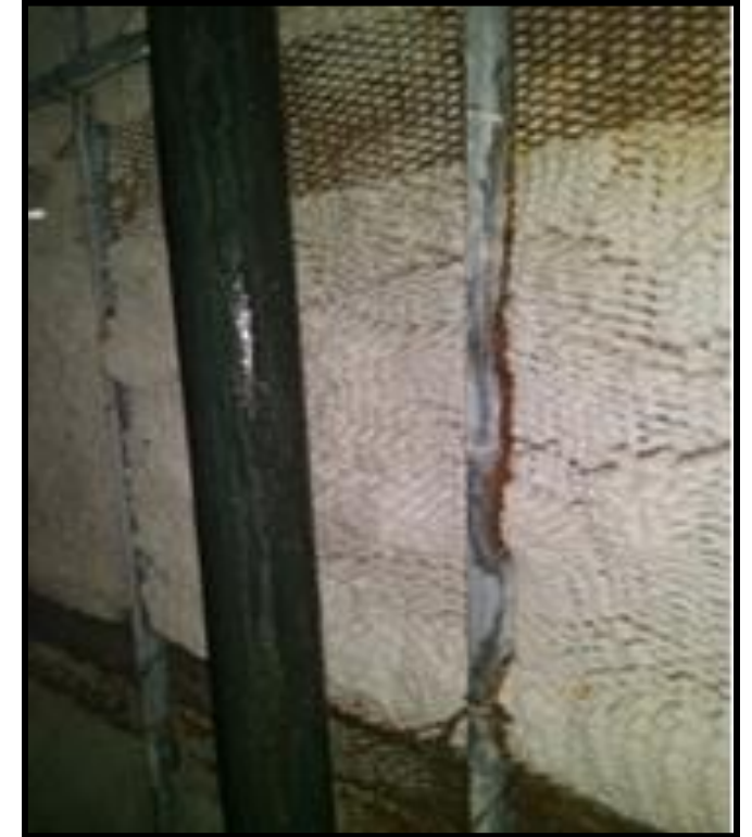
Example: condensation on the cold-water riser.
