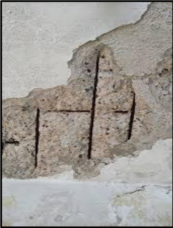
Photo #1: Exposed Rebar
