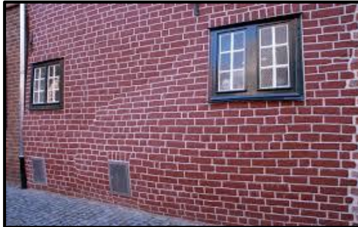
Photo #3: Bulging Wall
