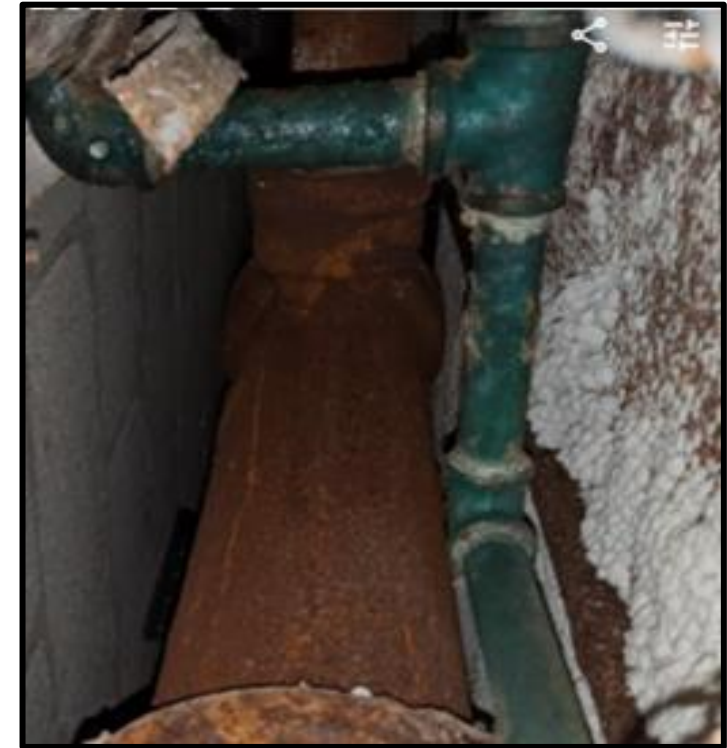
Example: Condensation on the cold-water supply pipes.
