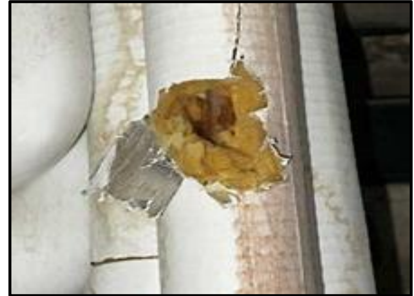
Example: torn pipe insulation.
